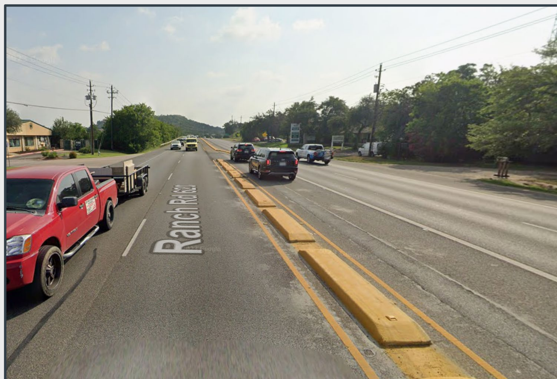
Median at Left-Turn Access
